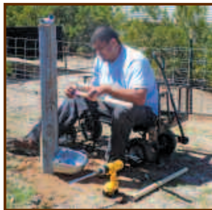
Lenny Plumbing a New Waterer
