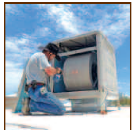
Jonny Repairing the B-Pen Cooler
